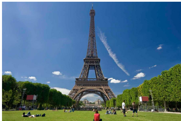
Figure 11. A 21 st century substation – completely invisible. The visual environmental impact is zero.
