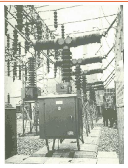
The photo shows two AEI 132kV Vacuum circuit Breakers which went into service in London with the CEGB in 1967 – 50 years ago!
