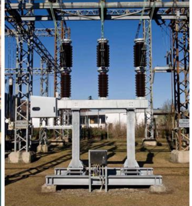
JAEPS 145kV Live Tank single break VCB on left with the Author and VI. On the right Siemens 72.5kV VCB
